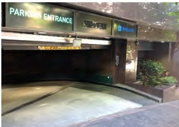
Parking garage with signed bike entrance over a delineated bike path (Photo: Alta Planning + Design)
