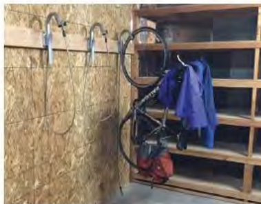
Anchoring and wood mounting is not theft resistant (Photo: MIG|SvR)
