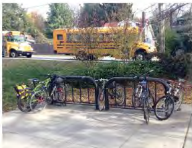
Rack does not allow use of a u-lock (Photo: Alta Planning + Design)
