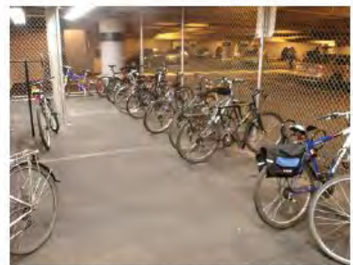
Racks do not provide 2 points of support (Photo: Alta Planning + Design)
