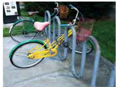
Rack does not provide 2 points of support (Photo: MIG|SvR)
