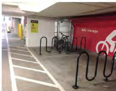
Racks do not provide 2 points of support & there is no delineated bike exit (Photo: Alta Planning + Design)
