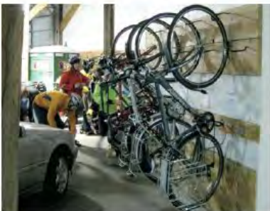
Anchoring is not theft resistant (Photo: MIG|SvR)
