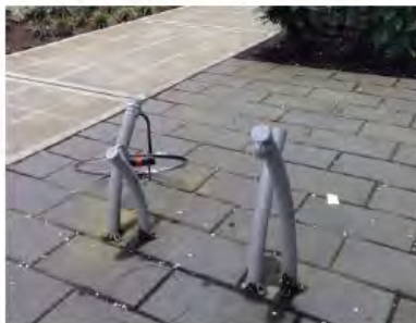
Non-intuitive rack does not provide 2 points of support (Photo: Alta Planning + Design)
